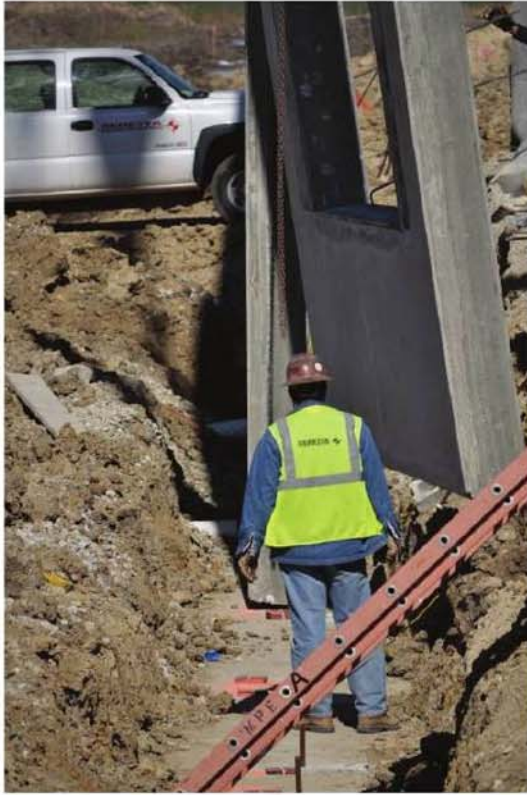
Tilt-up concrete panels are set on permanent, high-strength rectangular plastic shims. The shims create an open joint between the panel and the grade beam to receive grout, backer rod, and sealant.
